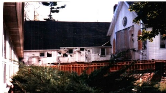
Preparation for construction & renovation (Gladys McEwan took various pictures, including these two.)
